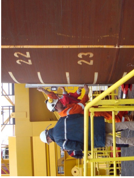
Along pile wall (Mini tilt)
