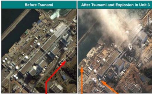
Before Tsunami After Tsunami and Explosion in Unit 3 Shared spent fuel pool building Missing heavy oil tanks Displaced oil tank?
