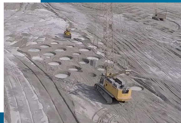
d) Backfilling operation. e) Start of the 1 st blow during the 2 nd pass. Execution of the required number of passes (2) .
