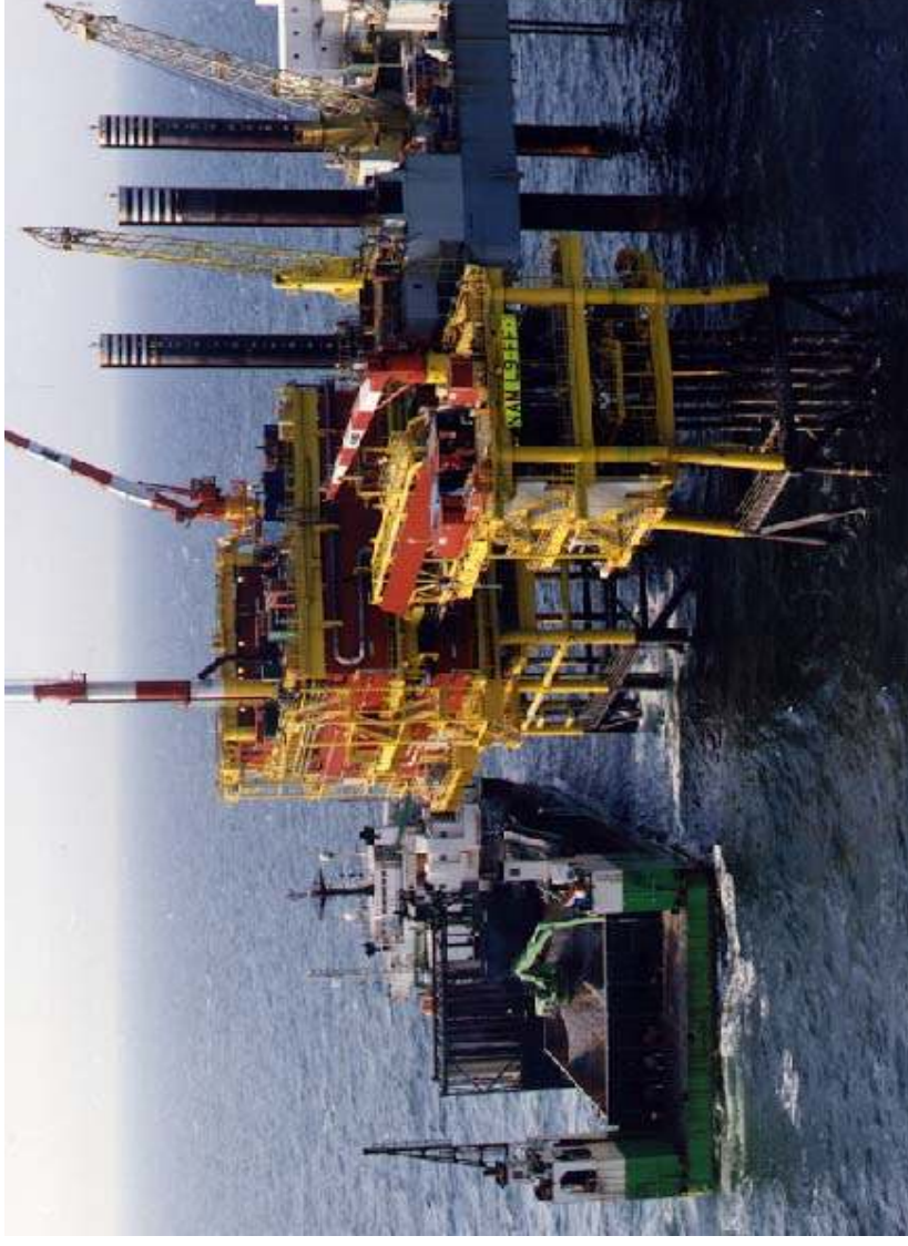
D.P. Fall Pipe Vessel "Rollingstone" - 11,500 tons
