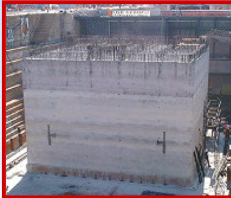
Concrete Gravity Base
