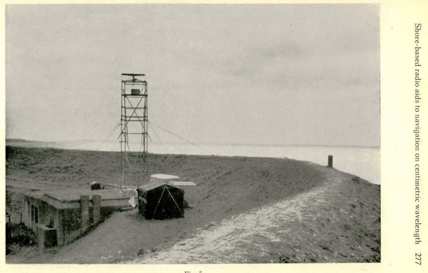
Fig. 3 Shore based radar equipment on mobile survey for the Scheldt estuary radar scheme
