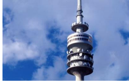
Operators wireless and broadcast networks
