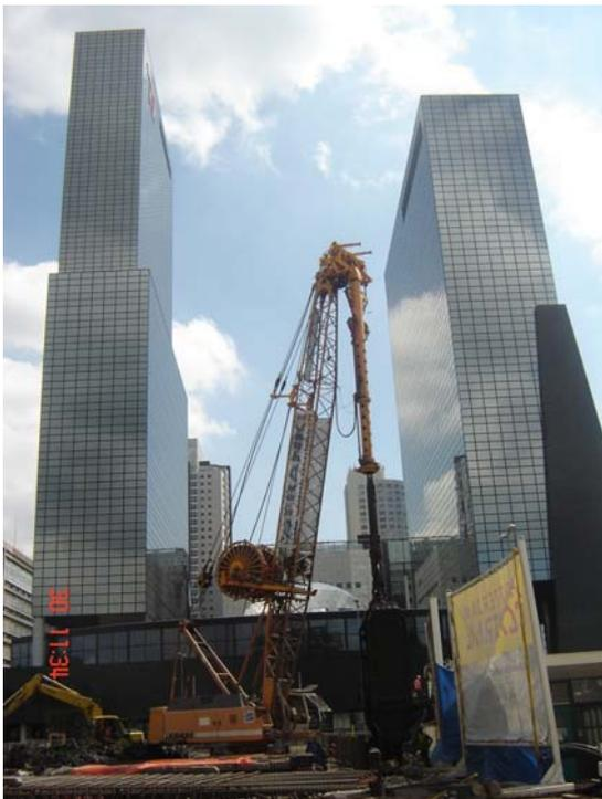
A total number of 100 freeze-pipes and temperature monitoring pipes were installed mainly vertically to a depth of ca. 40 m. Installation was done from the ground surface and from inside the underground tunnel. The ground freezing duration period was estimated to be at least 9 months.
