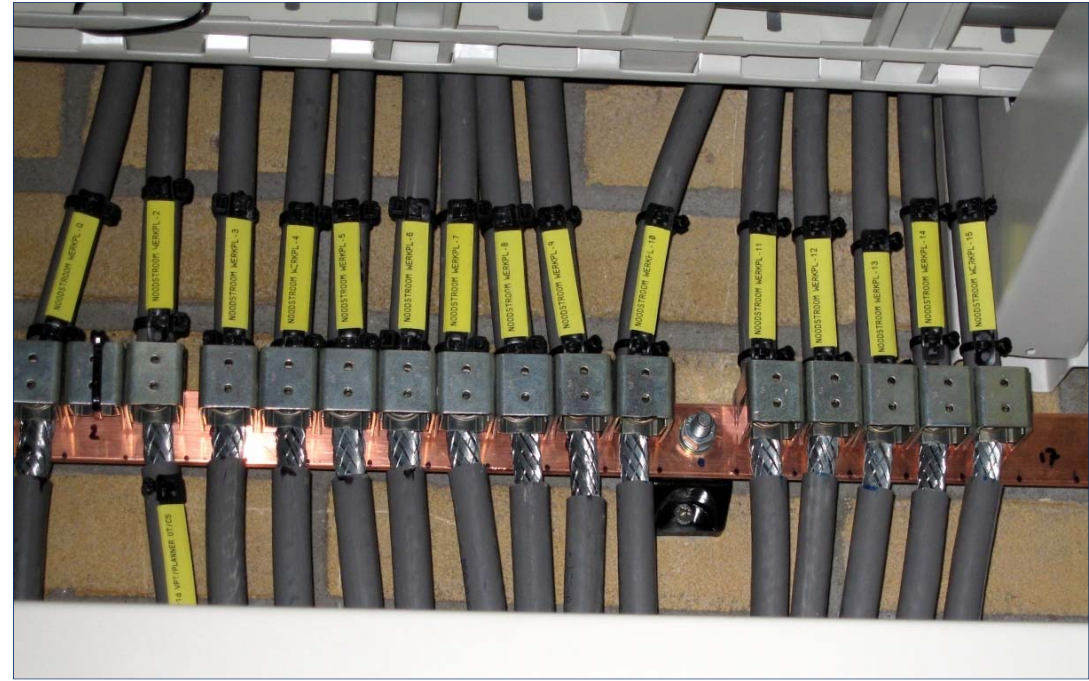
Shielding clamps at panel entry
