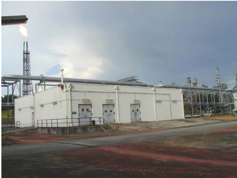
Control building of plant
