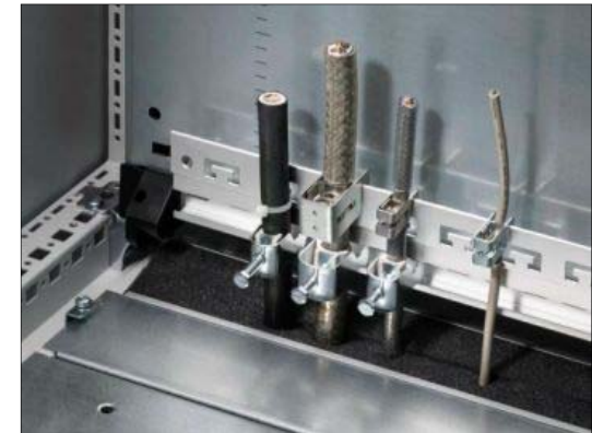
Shielding clamps at panel entry
