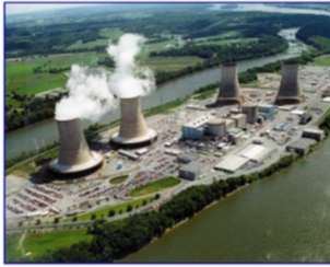
Three Mile Island, U.S.A., 03.28.1979, 4 a.m.
