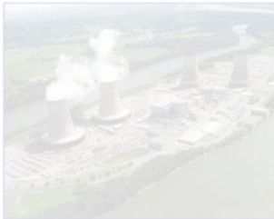
Three Mile Island, U.S.A., 03.28.1979, 4 a.m.
